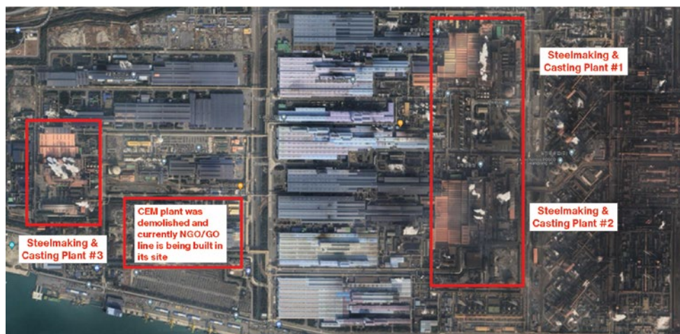
POSCO Gwangyang Works overview.
