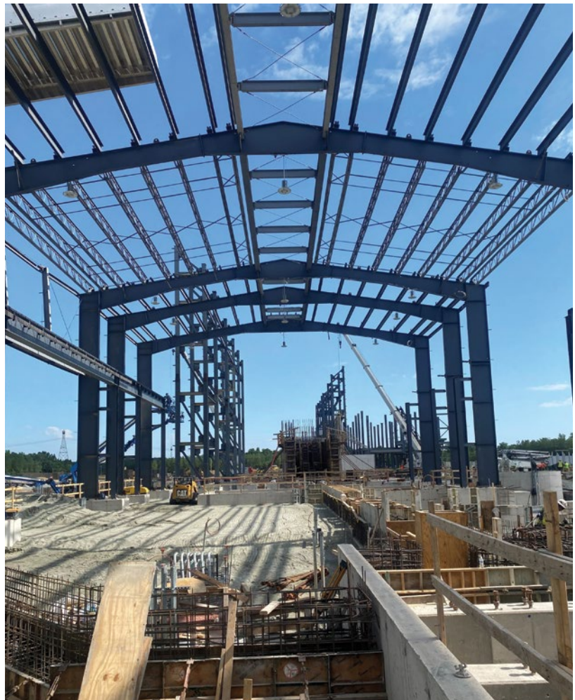
Construction image as of August 2024.
