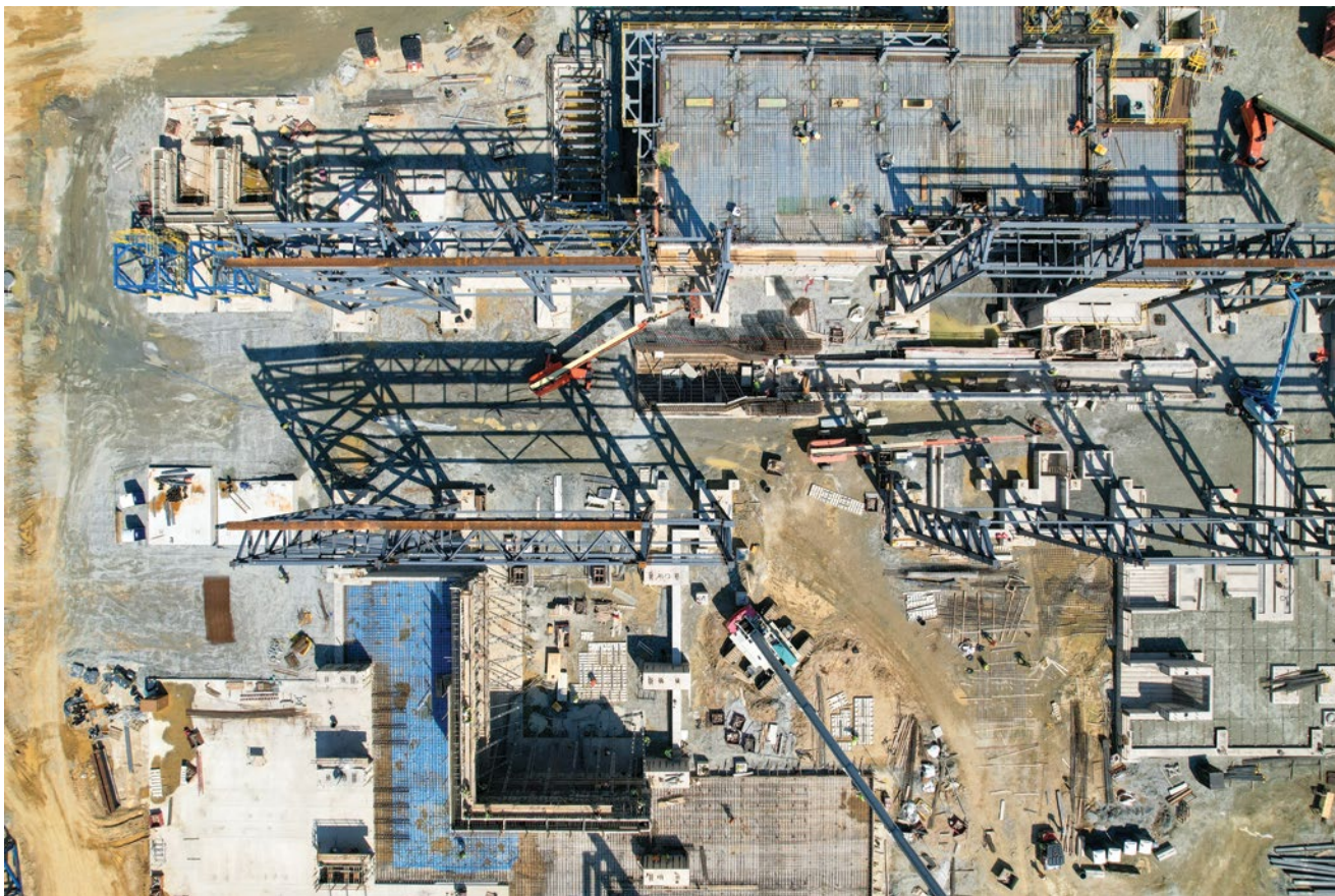
Construction image as of August 2024.
