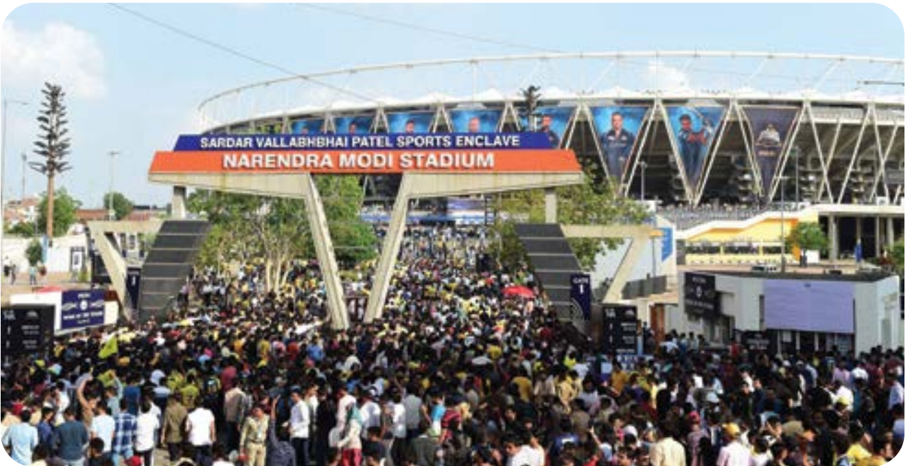
A ring of Y-shaped columns supports the world's largest cricket stadium. Photo by Populous.
